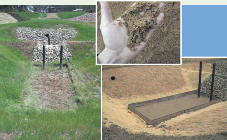
The coarse sand [center] used in this surface sand filter [left] provides physical and chemical water quality treatment. Erosion control matting protects the treatment after installation [right] until surrounding slopes are vegetated.
