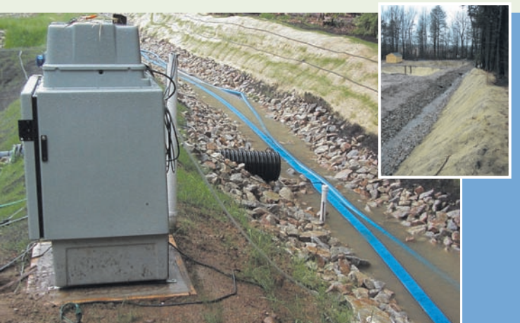
The stone swale [right] is designed to mimic a natural stream channel. Its combination of rock and fabric [left] helps trap sediment and promote vegetation. This treatment performed poorly for most evaluation criteria.
