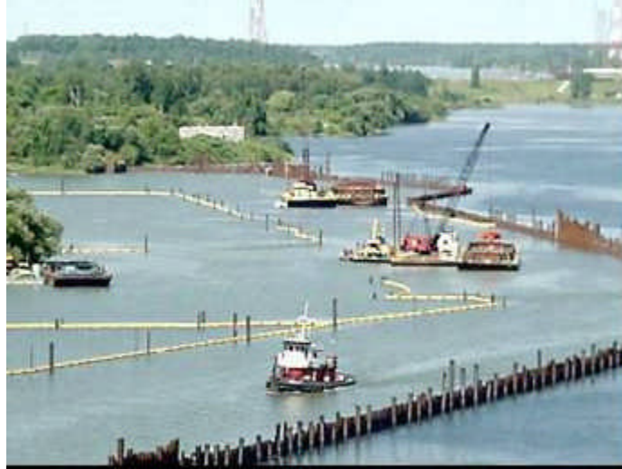
Figure 2-5. Fixed Sheet Piles
