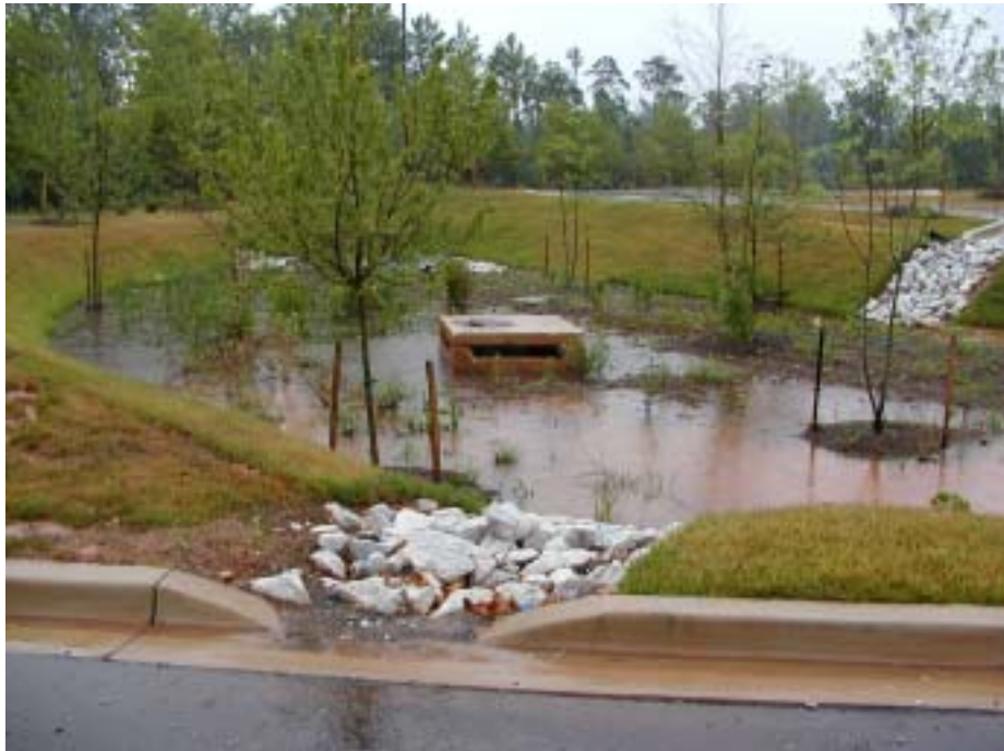
Figure 3. Collected Runoff through Curb-Cut during a Rain Event
