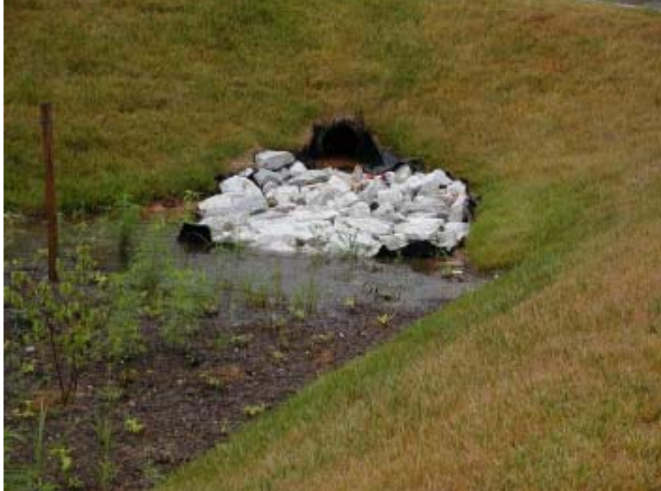
Figure 3. Collected Runoff through Curb-Cut during a Rain Event
